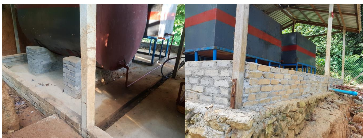
Figure (9) Containment walls for above ground fuel tanks
